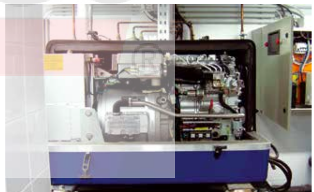
This three-phase Panda is installed in the basement. Main fuses, panel, and radiator control are fitted in electrical cabinet. Image: Kratos Kft. Hungary.
